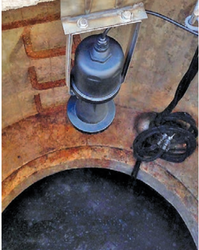
The LR30 pulse radar sensor is the reliable level measurement solution for municipal and industrial pump lift stations.
